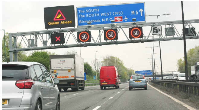
Fig. 1. A British highway equipped with 4 MSIs, where the left lane is closed and a temporary speed limit of 50 miles per hour is indicated on the other lanes. Image source: [5].
