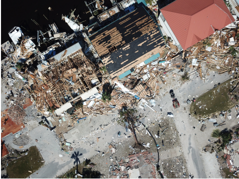
Fig. 1: Sample of Damage Scene from RescueNet. Buildings with different levels of damage as well as road parts.
