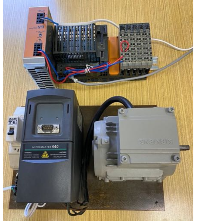
Fig. 6. Experimental setup of AC motor, inverter, and PLC.
