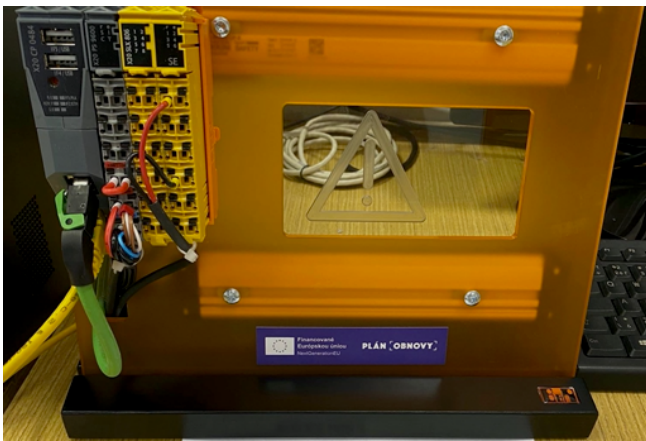
Fig. 5. Experimental setup for safety control with PLC.
