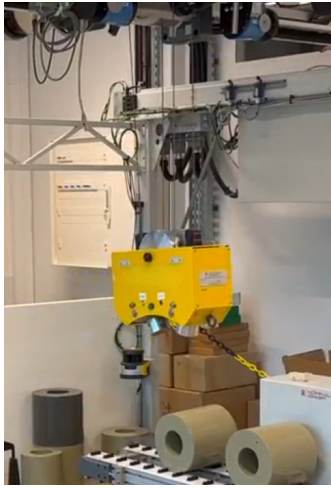
(a) Real overhead crane (unloaded case)
