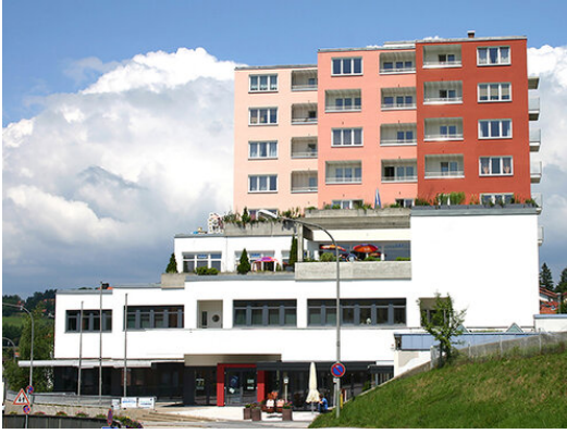
Fig. 6. The DIT building where the 5G measurements have been taken.
